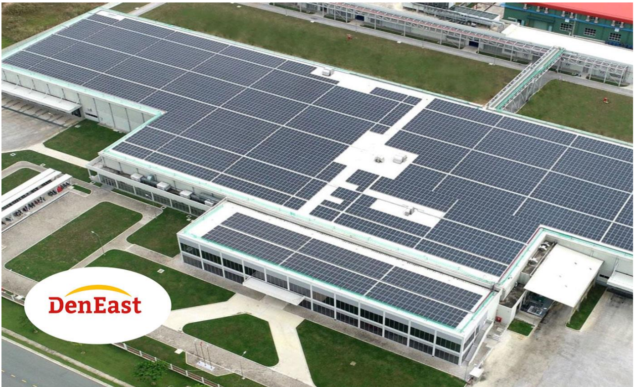
DenEast's ultra-modern aseptic packing plant is state-of-the-art.
